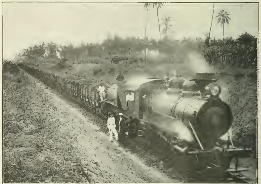
BALLAST TRAIN ON THE PHILIPPINE RAILWAY, CEBU, P. I.
